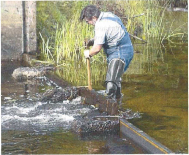
DNR maintenance specialist replacing wooden stop logs with steel channels at the Island Lake outlet dam in Crow Wing County (photograph by Ron and Judy Rolfe).
