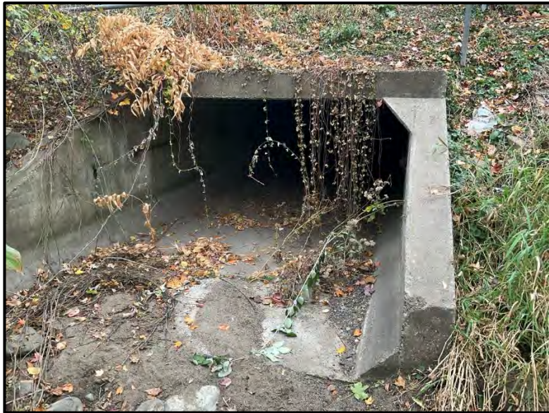
Markwood 8 feet x 4 feet Box Culvert (Crystal)
