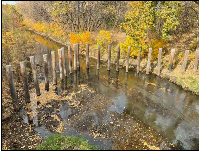
Debris Barrier (Minneapolis)
