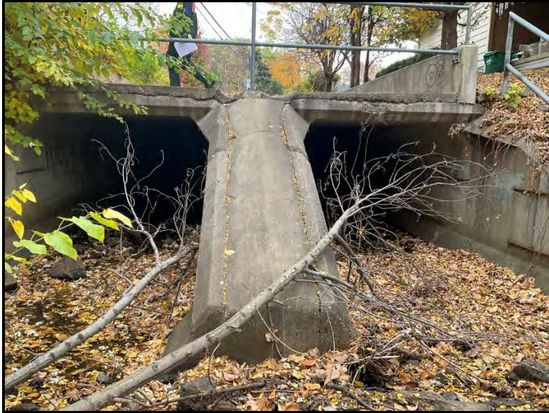
Markwood 8 feet x 4 feet Box Culvert (Crystal)
