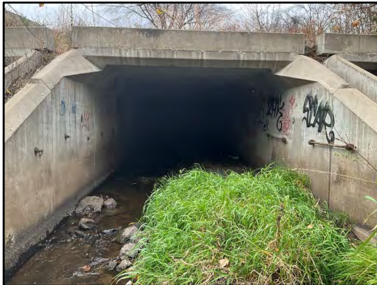
Highway 100 Double Box Culverts (MnDOT Responsibility, Located in Crystal/Golden Valley)
