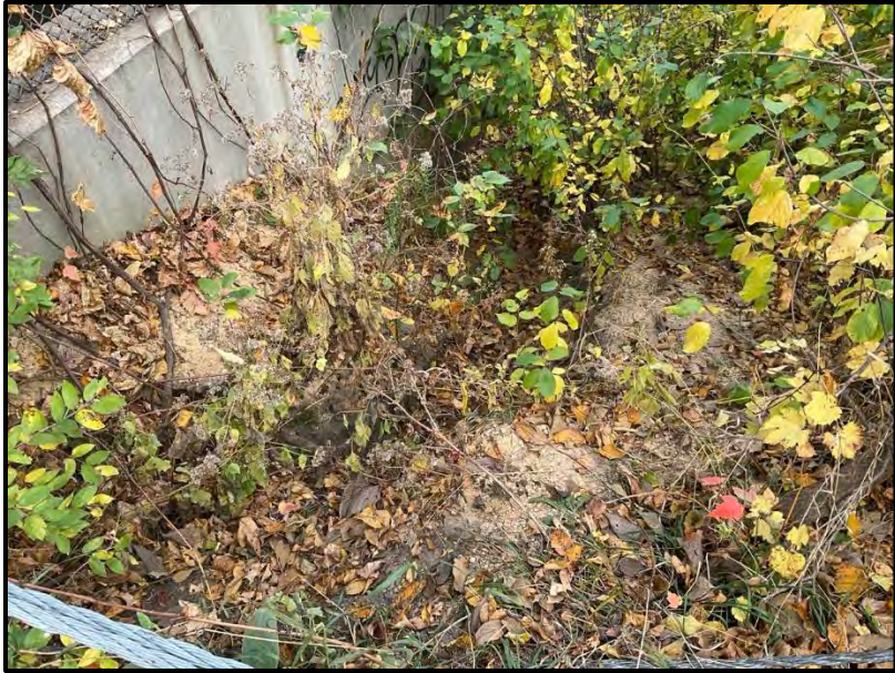
Highway 55 Control Structure (Golden Valley)
