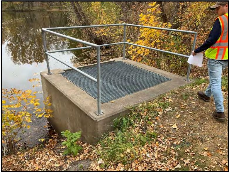
Detention Pond and Outlet Structure (Crystal)
