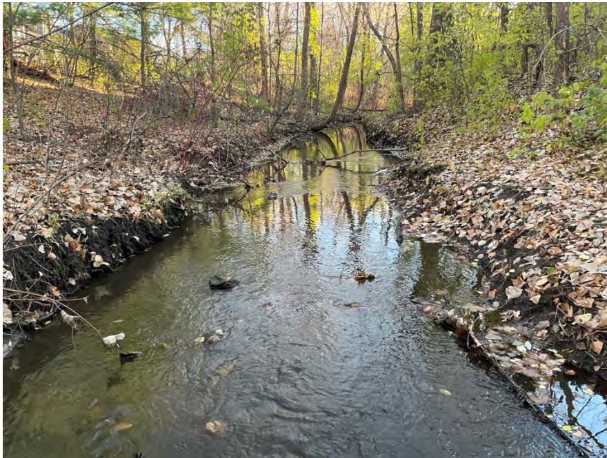
Photo 27: Site 3c. Looking downstream at station 42+90, both banks have minimal vegetative surface protection.
