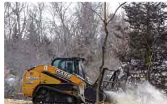
Example of Tree Removal: Forestry Mower Clearing Trees
