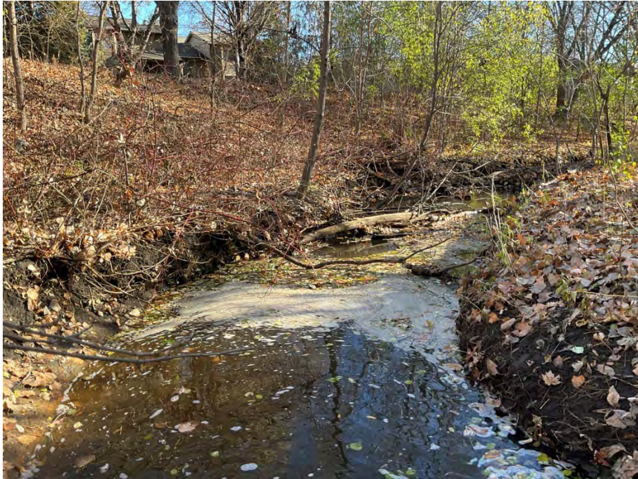
Photo 28: Site 3c. Looking downstream at a bend at station 45+20.
