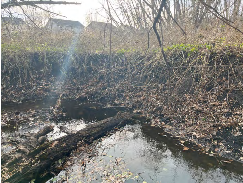
Photo 22: Site 2d. Looking at the right bank at station 27+90, the bank is mostly exposed.
