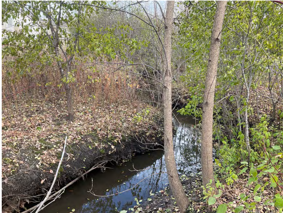
Photo 9: Site 1f. The creek begins to become more sinuous at station 11+40 and the left bank has undercut.
