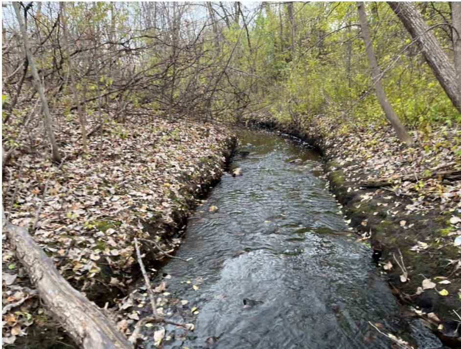
Photo 31: Site 4a. Looking downstream at station 54+00, downstream of the Rockford Road crossing. Undercut bank (six inches or less).
