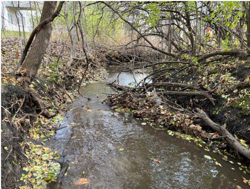
Photo 4: Site 1b. Looking downstream at station 5+00, both banks have tree roots present.
