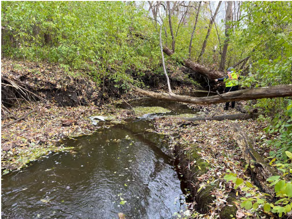
Photo 15: Site 2a. Looking downstream at station 19+20, this location is downstream of an outlet; flows with high exit velocities are eroding the left bank.
