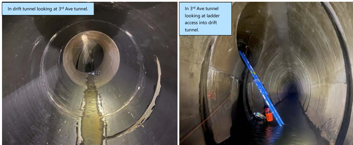
Figure 3-3 Drift Tunnel and Ladder Access
