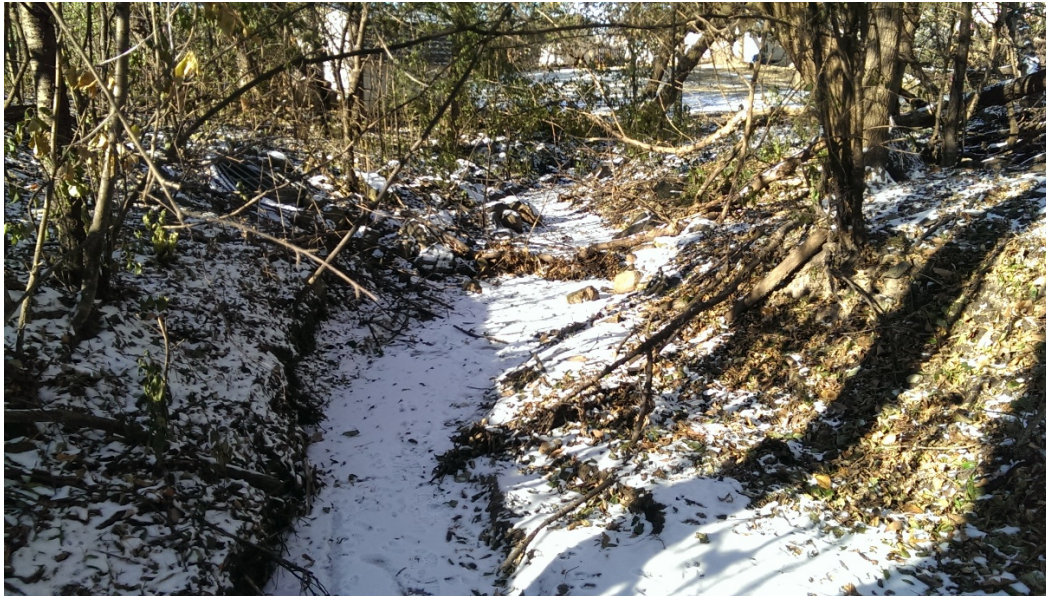
Figure 2 – Mt. Olivet, Reach 1, bank erosion
