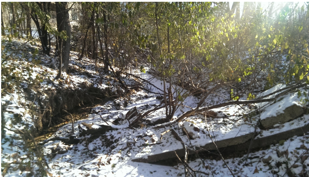
Figure 4 – Mt. Olivet, Reach 2, undercut bank and bank erosion cause by debris in stream channel
