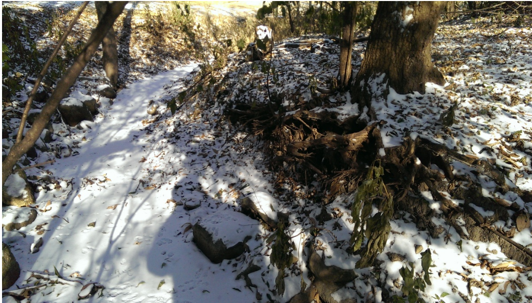
Figure 1 – Mt. Olivet, Reach 1, undercut bank erosion
