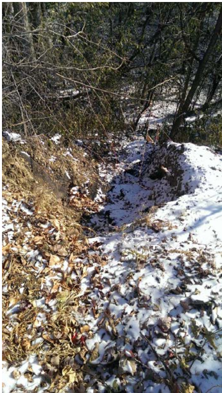
Figure 12 – Mt. Olivet, Reach 2, slope erosion from parking lot to the stream (view from above, same location as previous figure)
