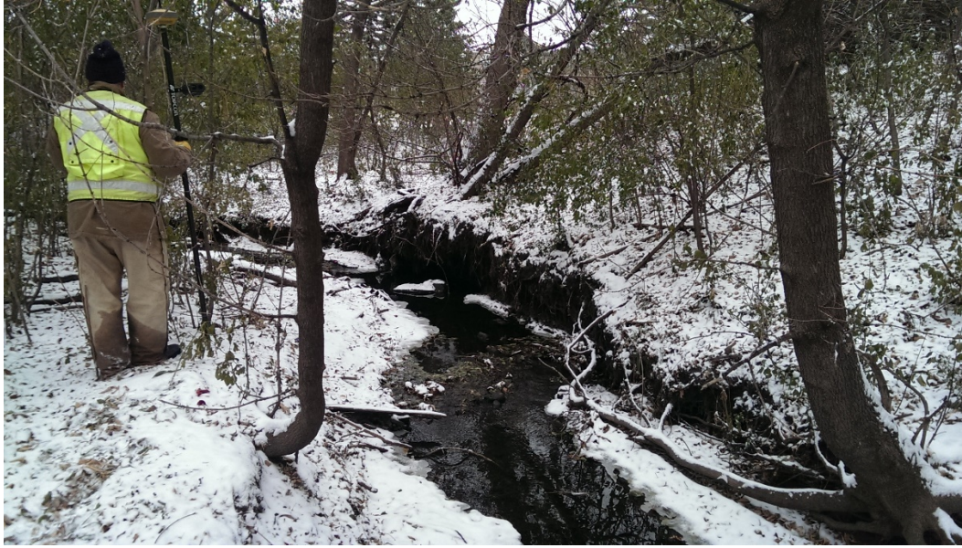
Figure 23 – Parkers Lake, Reach 1 bank scarp erosion
