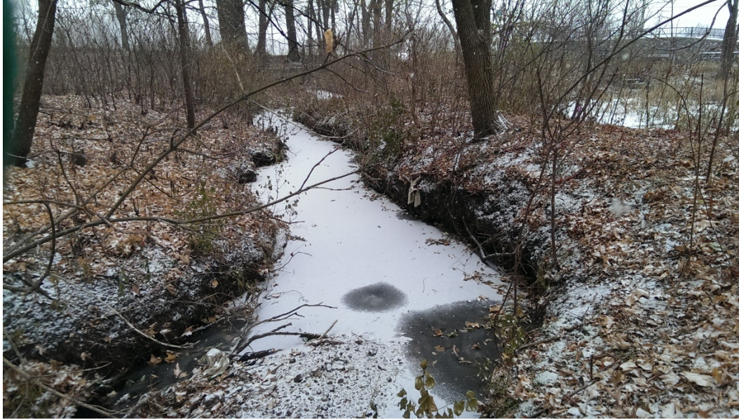
Figure 47 – Parkers Lake, Reach 2, undercut bank and bank erosion
