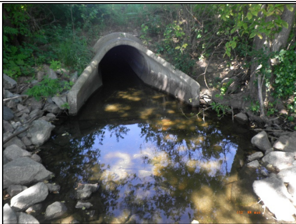
Photo 11: culvert located under the unnamed park access road.
