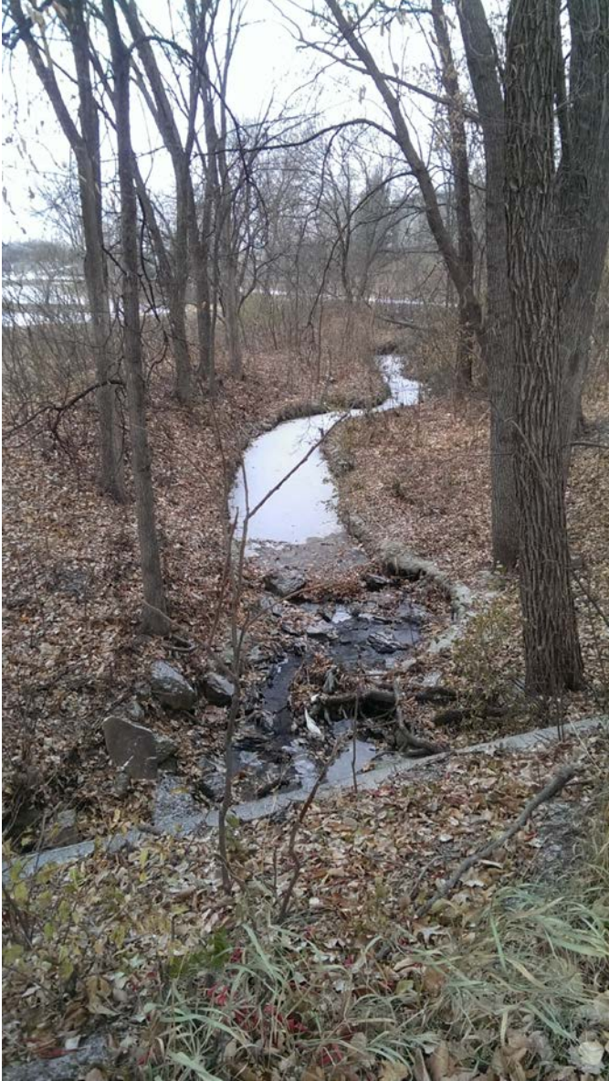
Figure 50 – Parkers Lake, Reach 2, bank erosion and head cut and bank erosion
