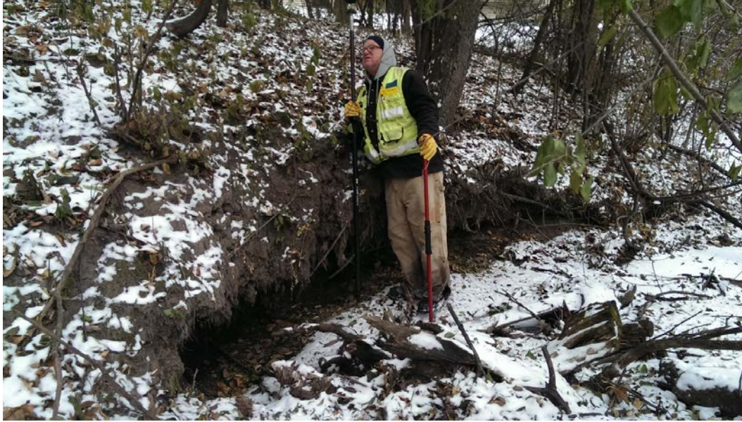
Figure 9 – Mt. Olivet, Reach 2, undercut bank and bank erosion cause by debris in channel
