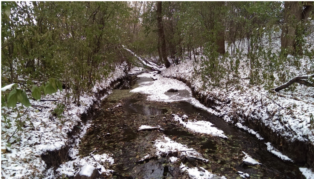
Figure 22 – Parkers Lake, Reach 1, bank erosion
