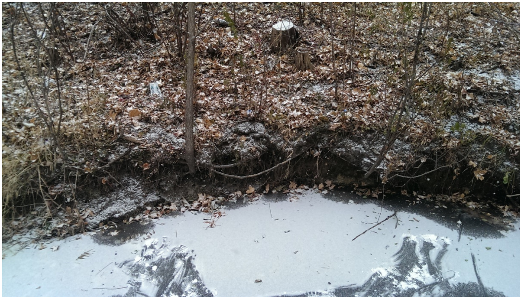
Figure 46 – Parkers Lake, Reach 2, undercut bank
