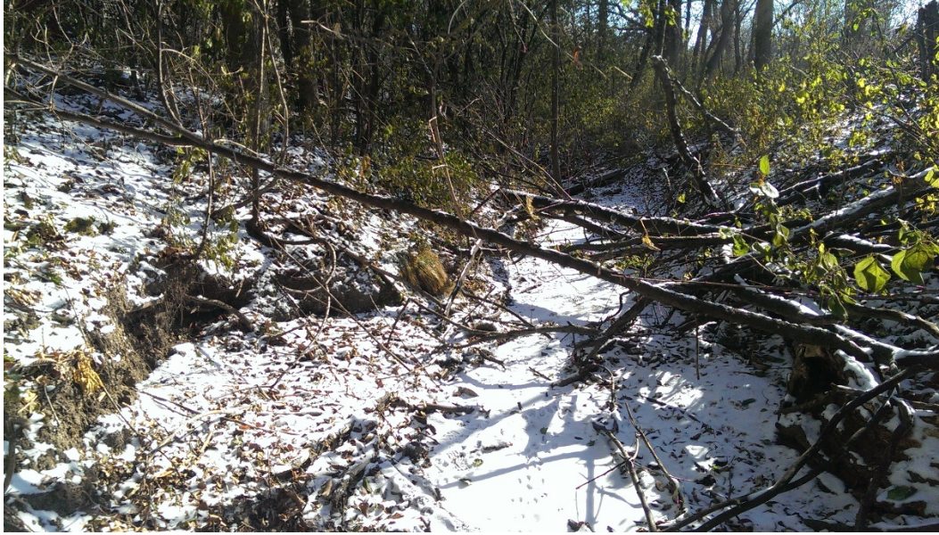
Figure 7 – Mt. Olivet, Reach 2, bank and channel erosion
