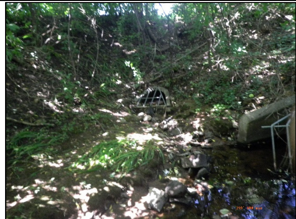
Photo 18: culvert located on the northern end of the project area.
