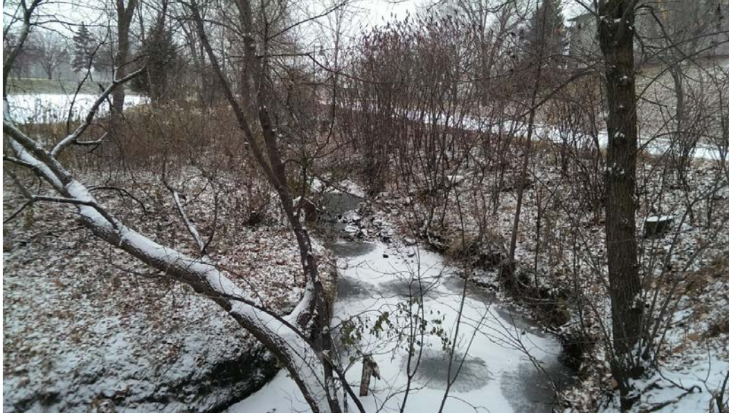
Figure 43 – Parkers Lake, Reach 2, undercut bank and bank erosion
