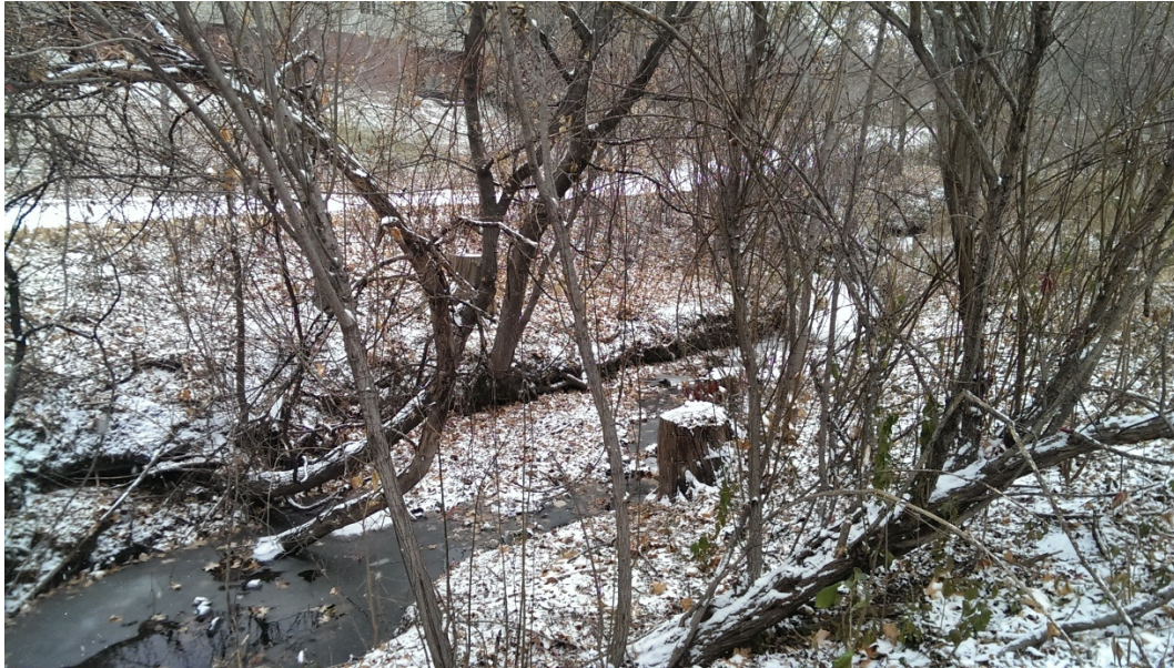
Figure 39 – Parkers Lake, Reach 2, bank erosion
