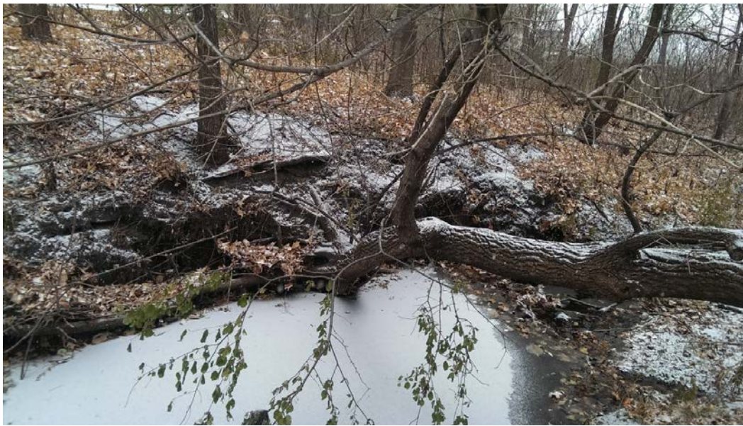
Figure 48 – Parkers Lake, Reach 2, undercut bank and scarp bank erosion
