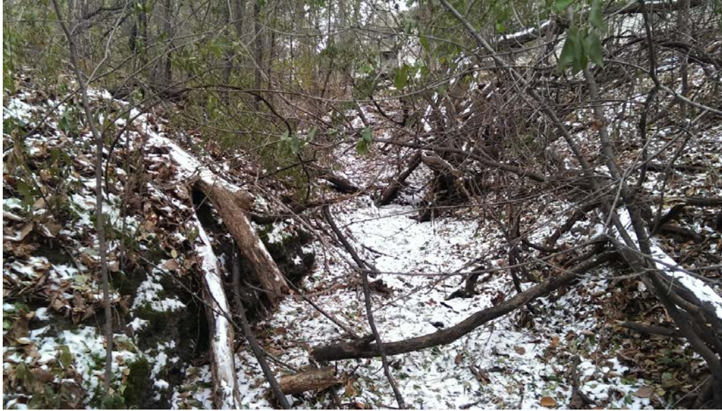
Figure 3 – Mt. Olivet, Reach 2, bank scarp erosion
