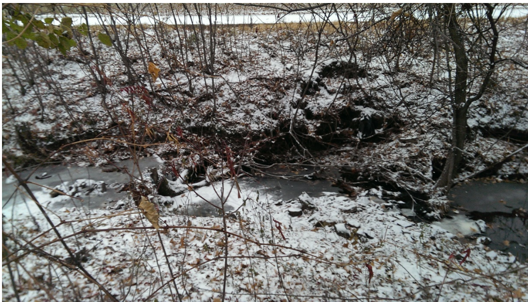
Figure 40 – Parkers Lake, Reach 2, bank scarp erosion
