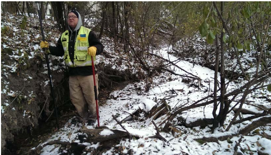
Figure 10 – Mt. Olivet, Reach 2, undercut bank and bank erosion cause by debris in channel (same location as previous figure)
