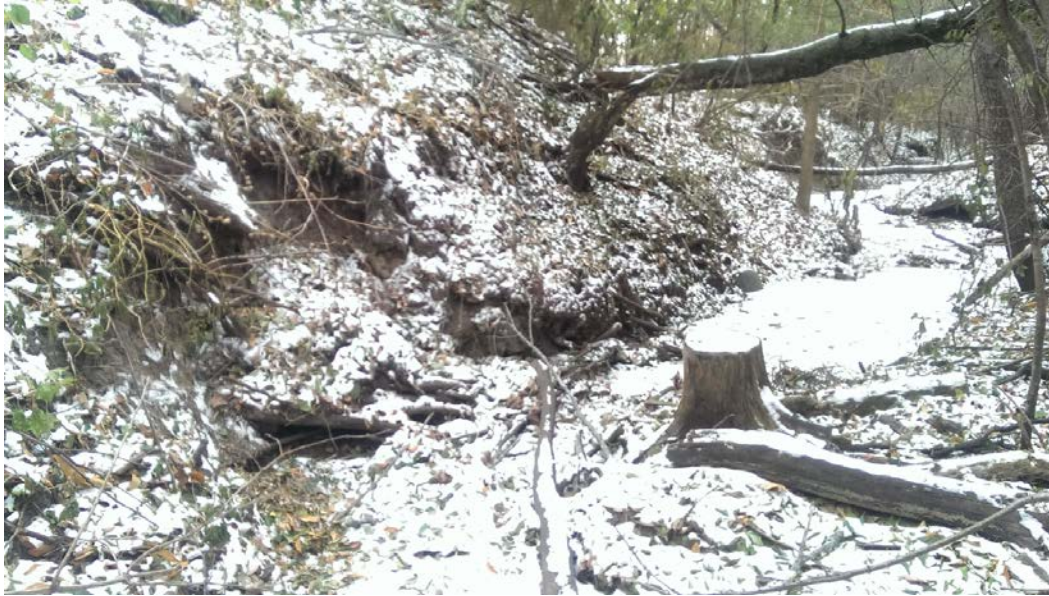
Figure 16 – Mt. Olivet, Reach 3, bank scarp erosion
