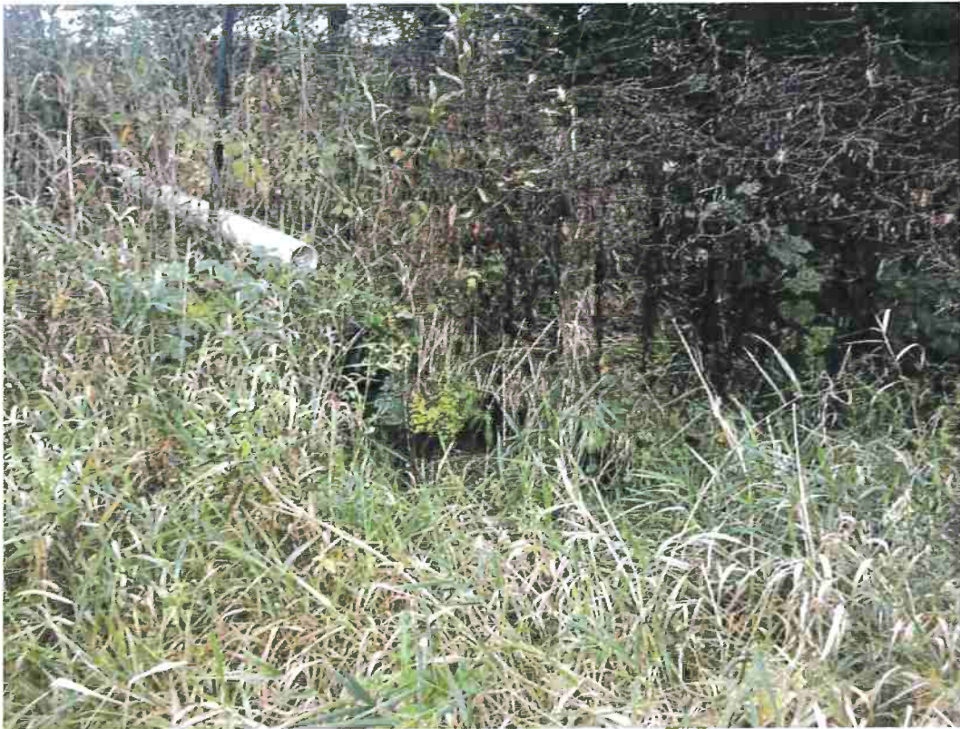
View of culvert draining from the south to Wetland 1.
