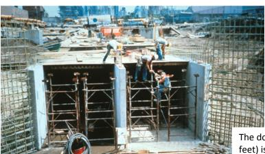
The double box culvert (each measuring 11x11 feet) is 1.1 miles long and was completed in 1992 by the Corps of Engineers.
