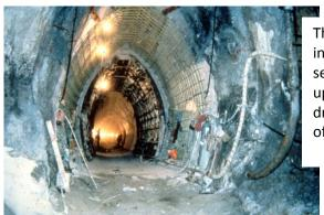
The Second Street tunnel, completed in 1978, is one mile in length with a 12-foot diameter equivalent arch. This section was constructed by MnDOT in a sandstone layer up to 80 feet below Second Street. It was designed to drain Interstates 394 and 94 along with parts of the City of Minneapolis and the Bassett Creek watershed.
