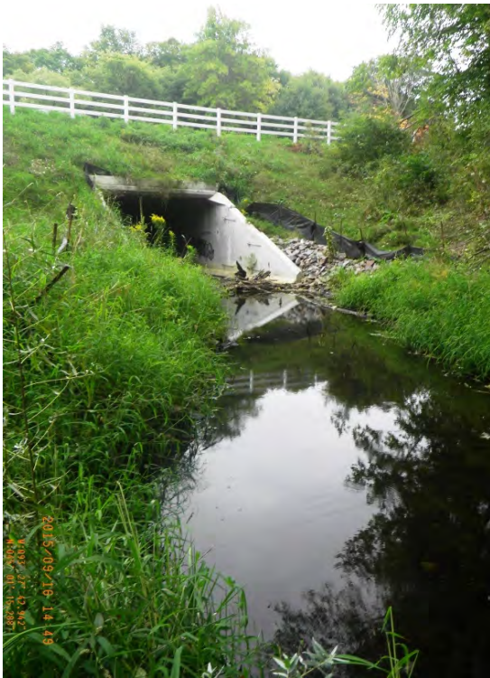
Photo 10: Culvert at Fernbrook Lane, looking southeast
