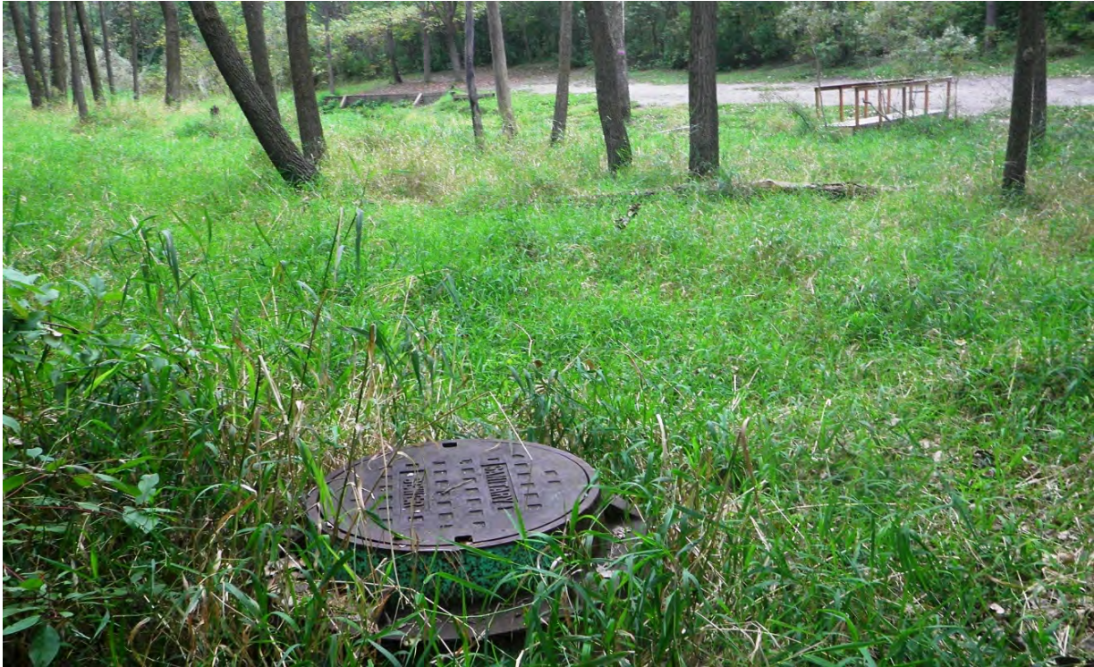
Photo 9: Sanitary sewer manhole, creek in background
