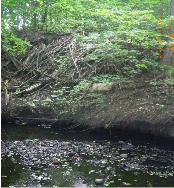
Photo 13: Debris (hot water heater, plastic, wood) in bank of creek east of Fernbrook Lane
