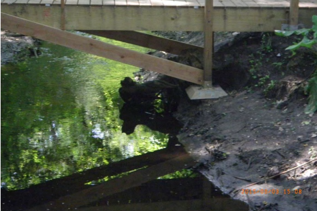
Photo 8. Site 9. Erosion around bridge abutments
