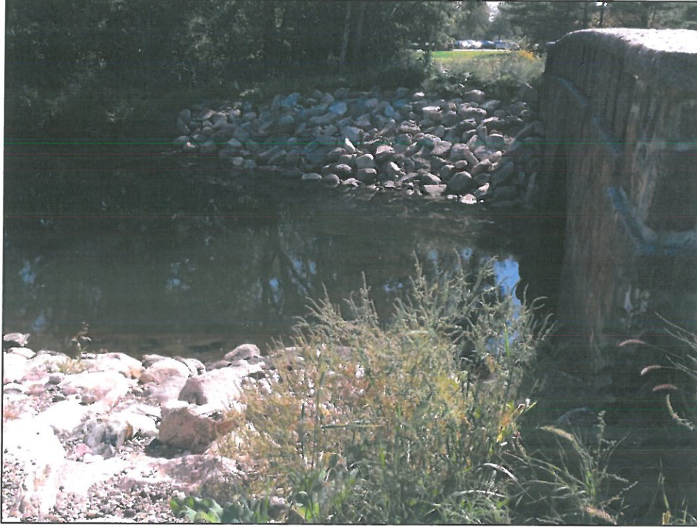
Site 4 – Parkway Bridge – 127+50 – AFTER
