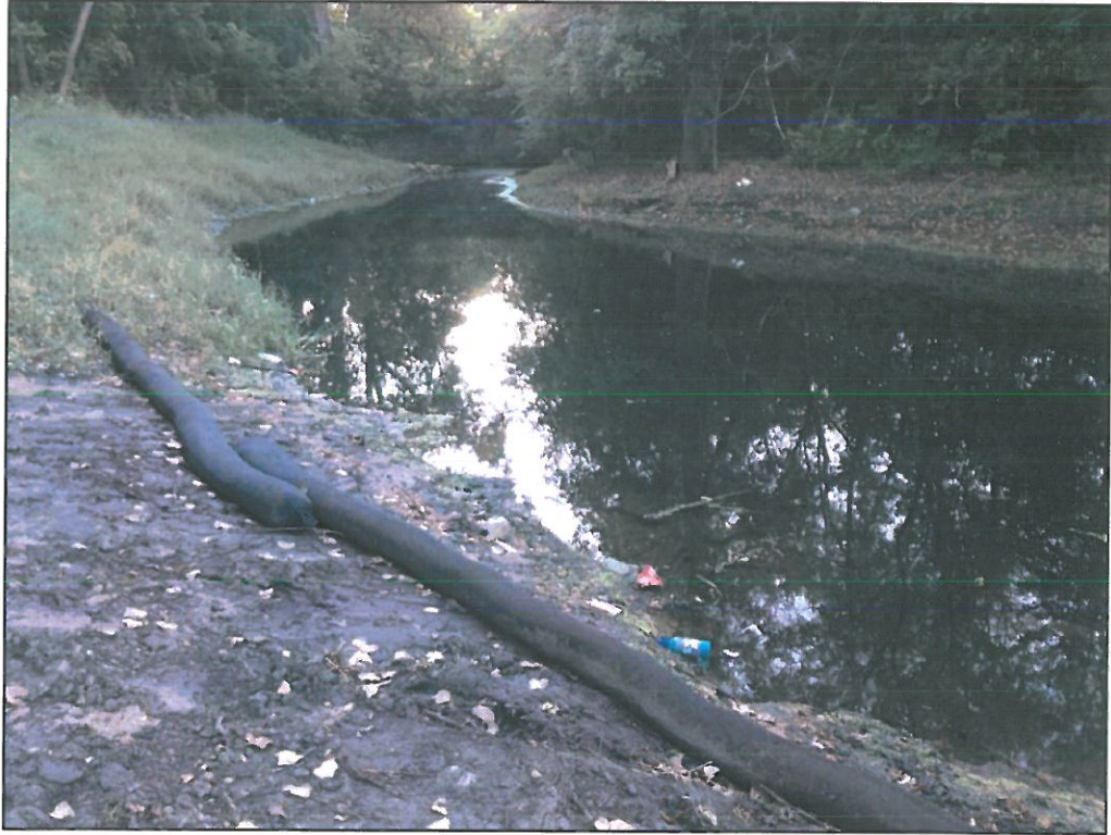
Bassett Creek Side Channel and Trail Work (work paid for by MPRB and city of Minneapolis) - AFTER
