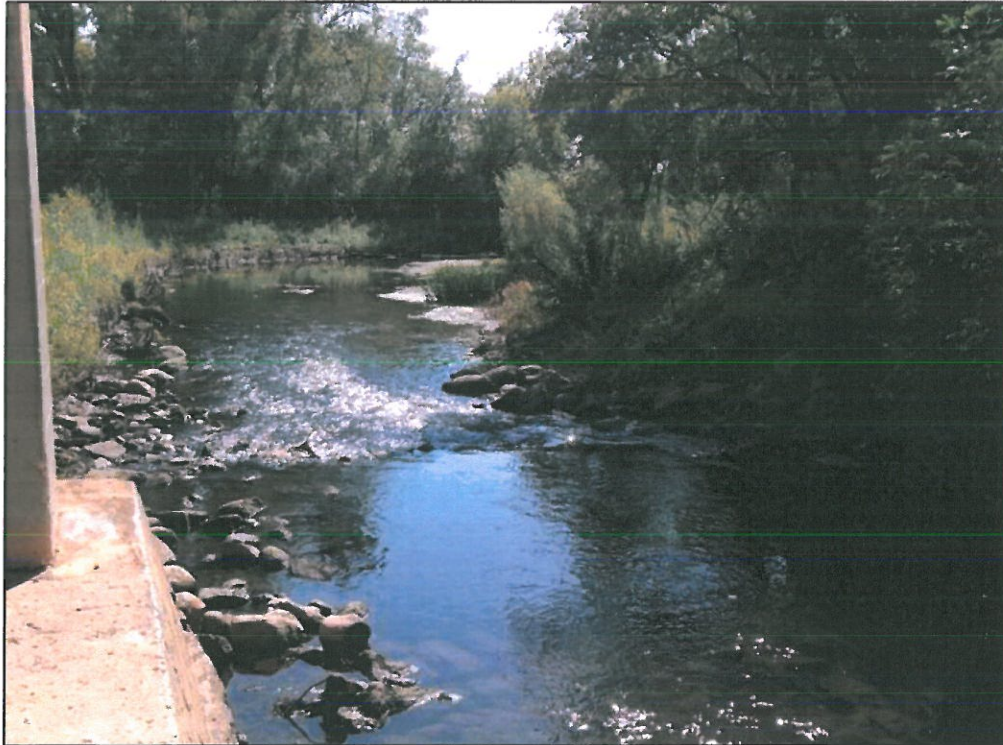
Site 4 – Parkway Bridge – 127+50 – AFTER
