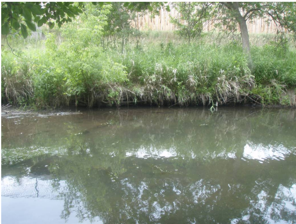
Photo 10. Site 10. Minor bank undercutting that could lead to future erosion.
